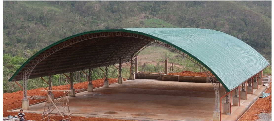
The completion of Open Gymnasium with project cost, PhP 2,598,979.30, at IFSU Aguineldo Campus was completed in November 2019.
