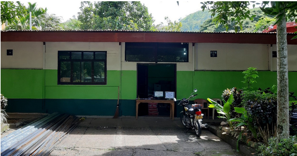
The improvement of the Supply Office at IFSU Lamut Campus with project cost, PhP 355,000, was completed in October 2019
