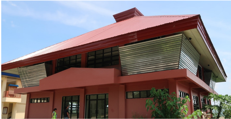
The replacement of the Library Building with project cost, PhP 1,488,379.67, at IFSU Potia Campus was completed in January 2019.
