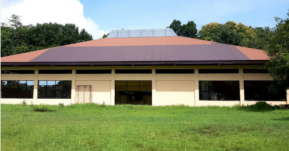
The Covered Court & Bleachers for Physical Education Faculty & Teachers at IFSU Lamut Campus with project cost, PhP 14,699,047.05, was completed in January 2019
